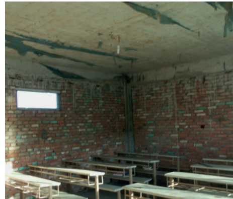
Before the renovations, there were no windows or plaster on the walls & ceilings.
